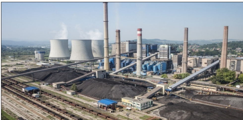
Fig. 2: Thermal power plant „Tuzla“ in Tuzla Source: Electric Power Industry of Bosnia and Herzegovina, 2019.
